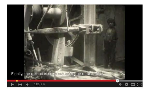
Text: Finally, the drill bit is spun out using the rotary table.
