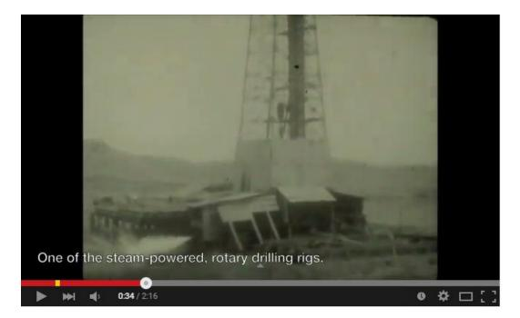
**Text:** One of the steam-powered, rotary drilling rigs.
