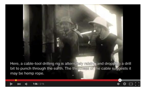
**Text:** Here, a cable-tool drilling rig is alternately raising and dropping a drill bit to punch through the earth. The thickness of the cable suggests it may be hemp rope.
