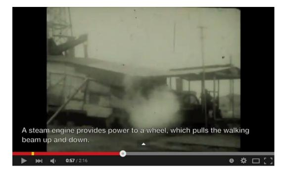
Text: A steam engine provides power to a wheel, which pulls the walking beam up and down.
