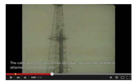
**Text:** The cable pulls sections of five-inch pipe, to which the drill bit is attached, out of the oil well.
