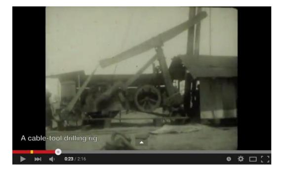
Text: A cable-tool drilling rig.
